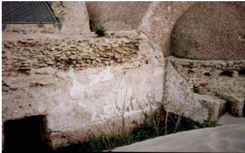
Fig. 9.6 Sokkelzone in Leptis Magna
